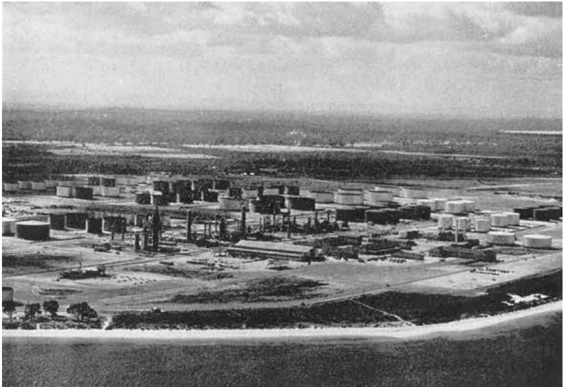
FIGURE 3. THE ANGLO-IRANIAN OIL COMPANY REFINERY NEARING COMPLETION
