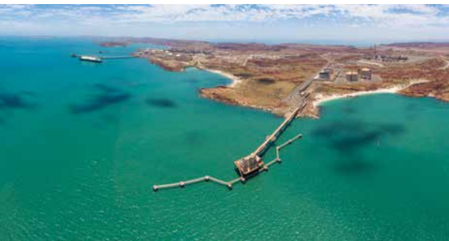
Pluto LNG Onshore Gas Plant and Loading Jetty. Source: Courtesy of Woodside Energy Ltd.
