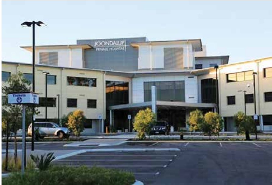
Joondalup Health Campus. Source: Project Directors Australia, 2017.
