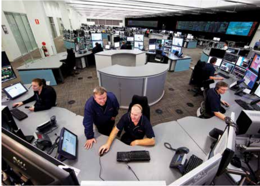
Rio Tinto's Operations Centre, Perth. Source: Courtesy of Rio Tinto.
