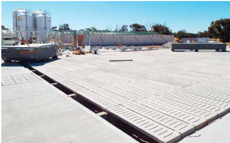
GD Pork Facilities. Source: Finrone Systems, 2017.
