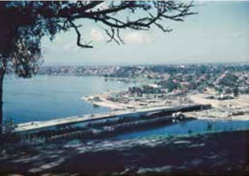
The Narrows Bridge in its final stages of construction, 1959. Source: Wylie 1959.
