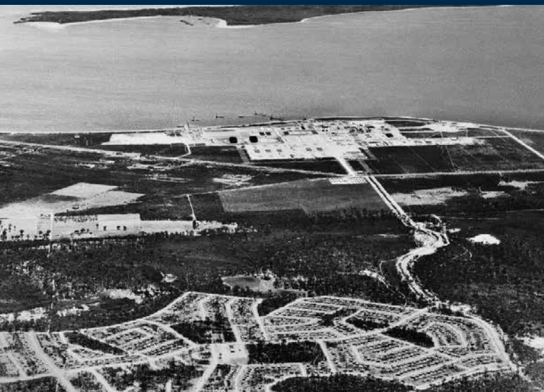
BP Refinery, Kwinana. Source: Courtesy of BP Development Australia Pty Ltd.
