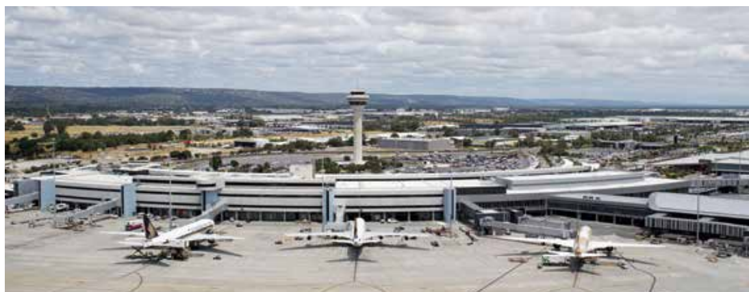
Perth Airport T1. Source: Courtesy of Perth Airport Pty Ltd.
