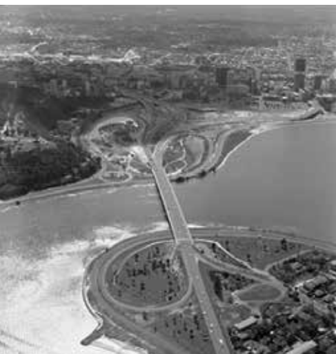
The Narrows Bridge, connecting the north and south metropolitan areas. Source: Stevenson, Kinder & Scott Corporate Photography, 1974.
